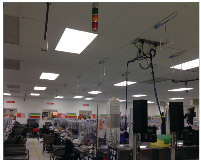
Ceiling Emitters in Production
